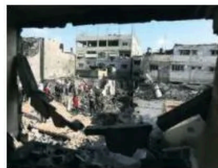
A damaged building after an Israeli airstrike on Khan Younis in Gaza on Dec. 1, 2023. The New York Times
